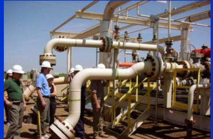
Main CO 2 pipeline enters Weyburn
